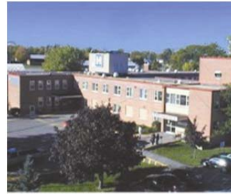
QHC Prince Edward County Memorial Hospital
